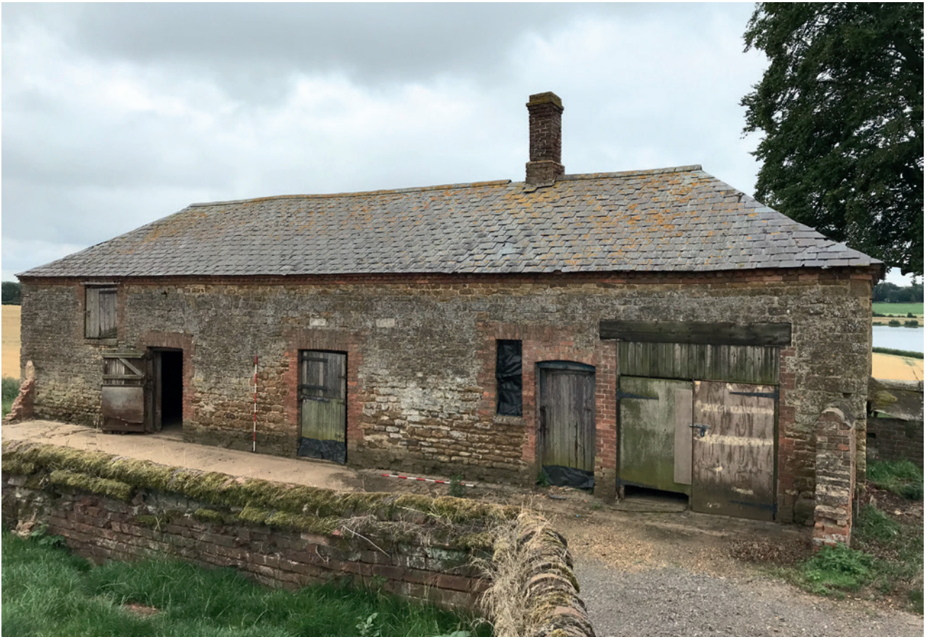
Figure 13: The coach house and stable block, Grange Farm, Holcot Road, Brixworth
