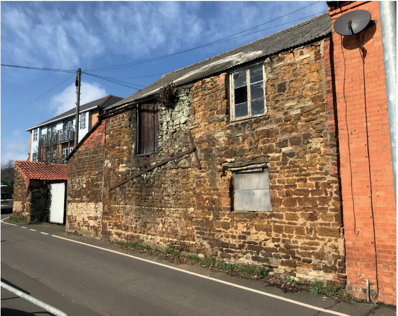
Figure 21: Jackson's Lane, Wellingborough. A probable 18th century dwelling converted to a barn, cart shed and stable in the 19th century
