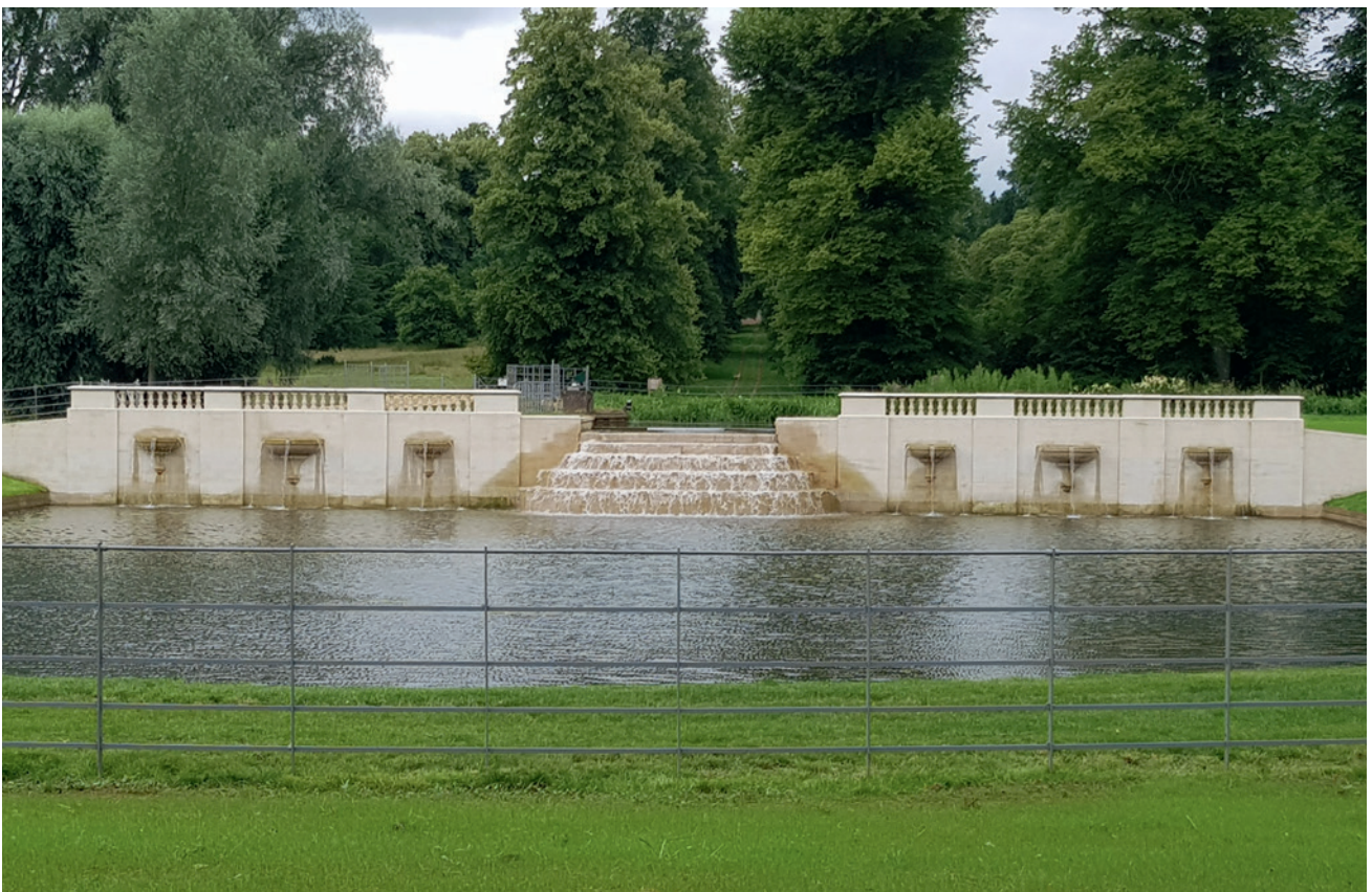
Figure 12 Boughton House, Star Pond with reconstructed facade and cascade: Liz Mordue
