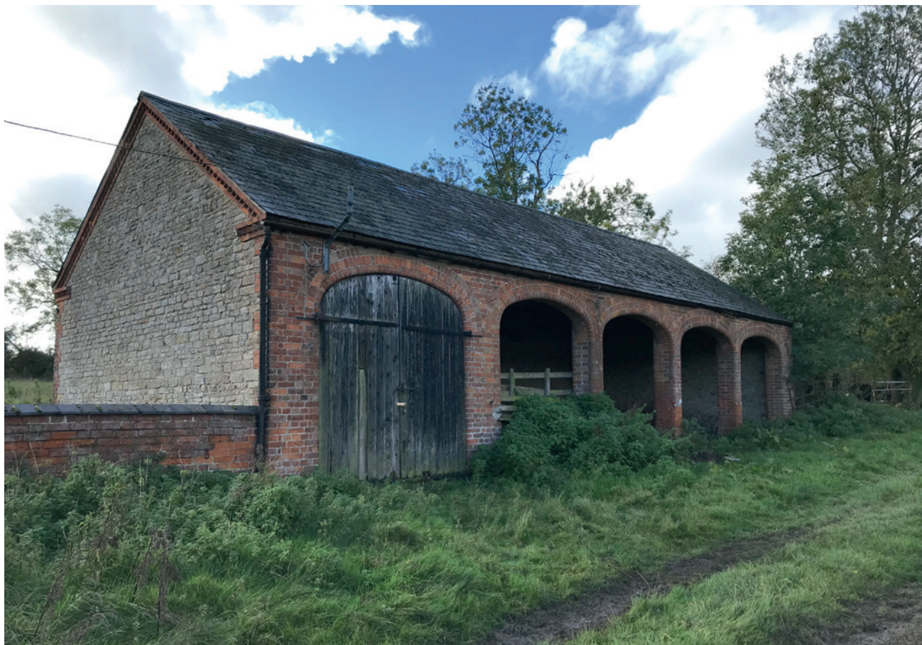
Figure 23: Cart and implement shed, built in 1878, Elderswell Farm, Turvey
